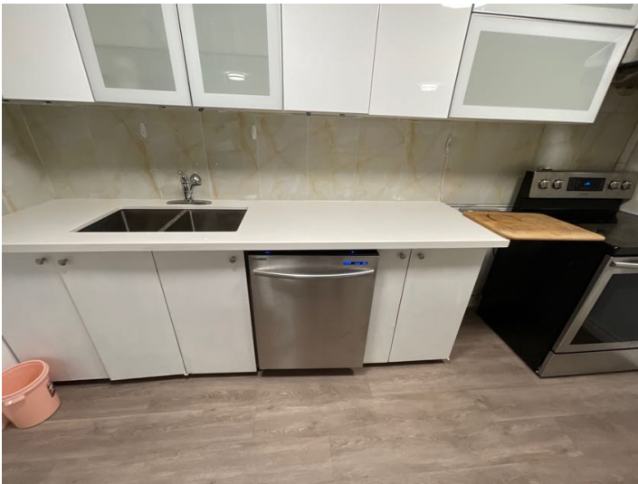
There are no electrical outlets on the countertop area.
