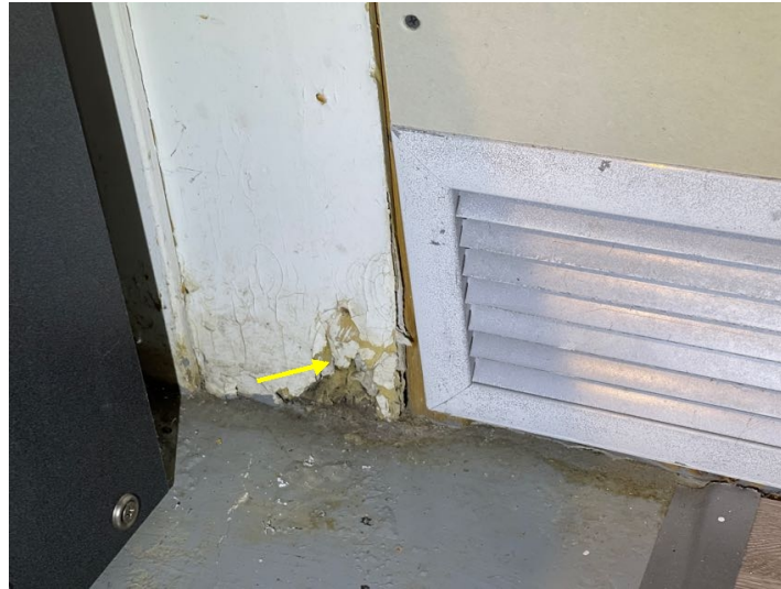
G next to the laundry room entrance door
